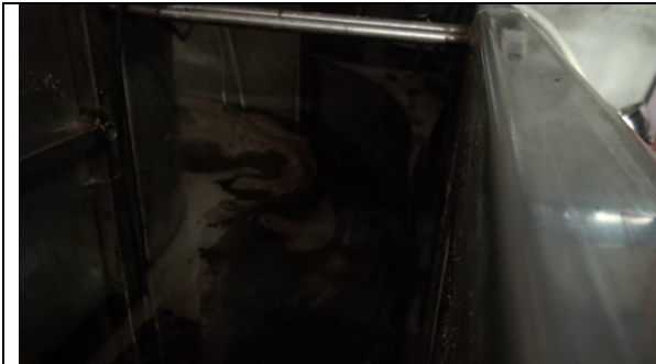
Figure C-o-109: CLB R 4 S 1 Oil migrating around tank
