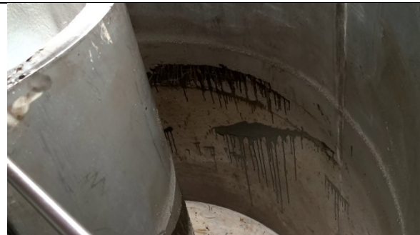
Figure C-o-142: HFO R3 S5 Cleanup
