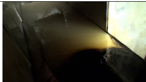
Figure C-o-104 CLB R 3 S 3 Oil hold-up between window and thruster
