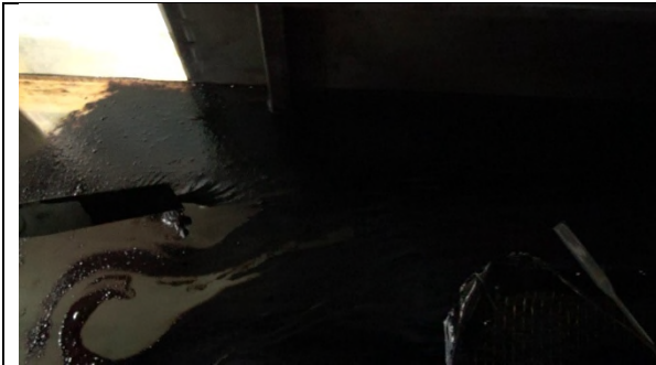
Figure C-o-74: CHV R2 S10 Oil hold-up from chiller to thrusters
