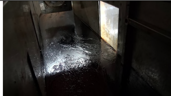
Figure C-o-62: AWB R4 S6 Hold-up under fan
