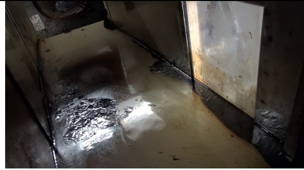
Figure C-o-18 AHS R4 S7 Oil losses from surface are apparent
