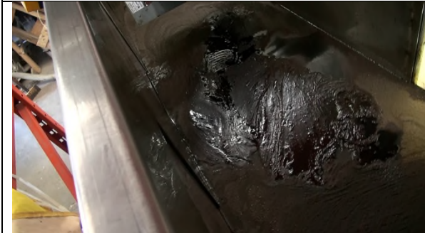
Figure C-o-296: WCS R1 S8 Hold-up on N side
