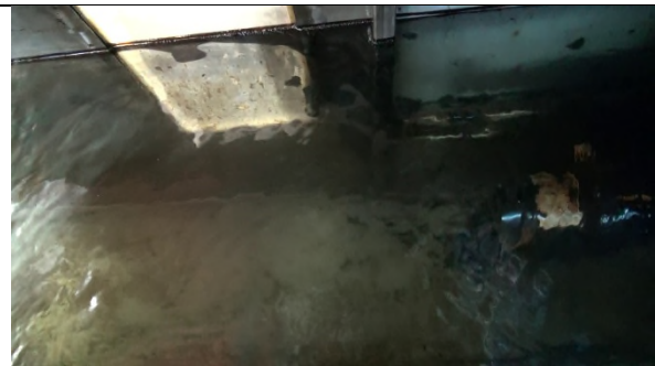
Figure C-o-4 AHS R 1 S 5 Bulk oil had effectively sunken by S 5
