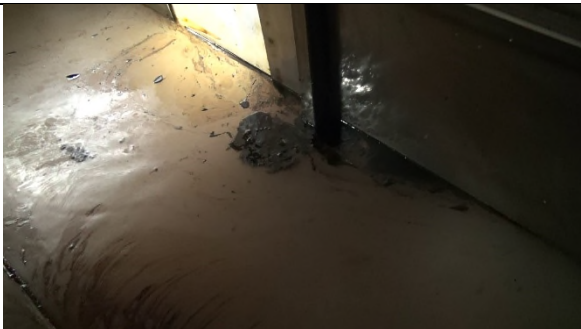
Figure C-o-141: HFO R3 S2 Little oil remaining at surface
